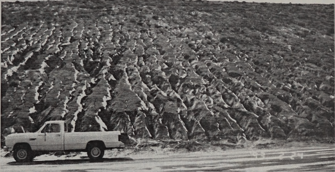
Figure 2: Example of accelerated erosional processes and mass movement on a small scale due to road construction.
